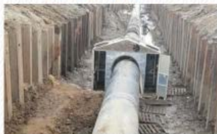
TANAP & TAP Tie-in, Greece
