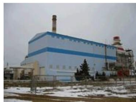
Shimal power station (1 st unit)
