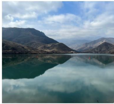
Sugovushan Water Reservoir
