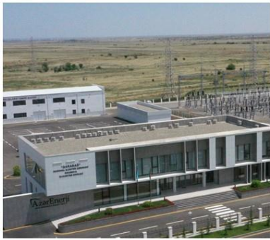
AzerEnergy Karabakh Regional Digital Control Center
