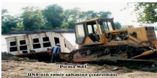
Piraza MIU - Taking the FPS to the repair site
