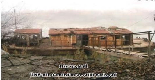
Piraza MIU - Condition of FPS before repair
