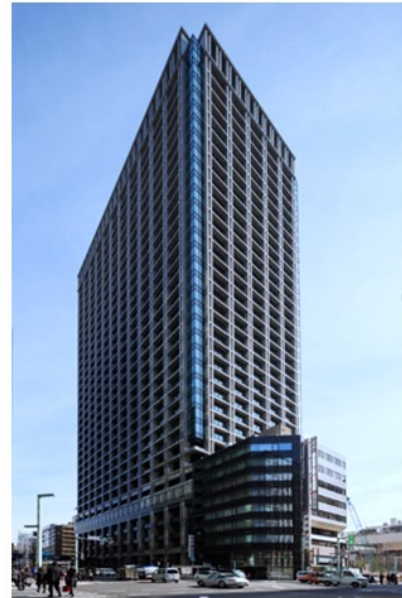
Marubeni Head Office, Tokyo
