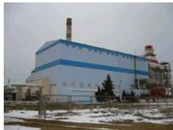
Shimal power station (loan, 1998, 1999)
