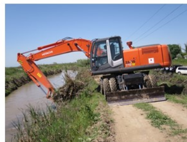
Procured excavator (Grant, 2013)
